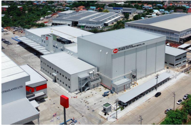
[Exterior View of the New Warehouse]
